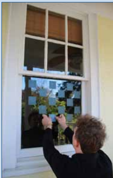
Window tape patterns are easy to apply and provide an effective deterrent against bird strikes. Shown is ABC Bird Tape. Photo: Dariusz Zdziebkowski, ABC.
